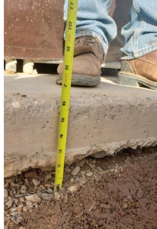
Figure 7: Measurement of slab thickness
